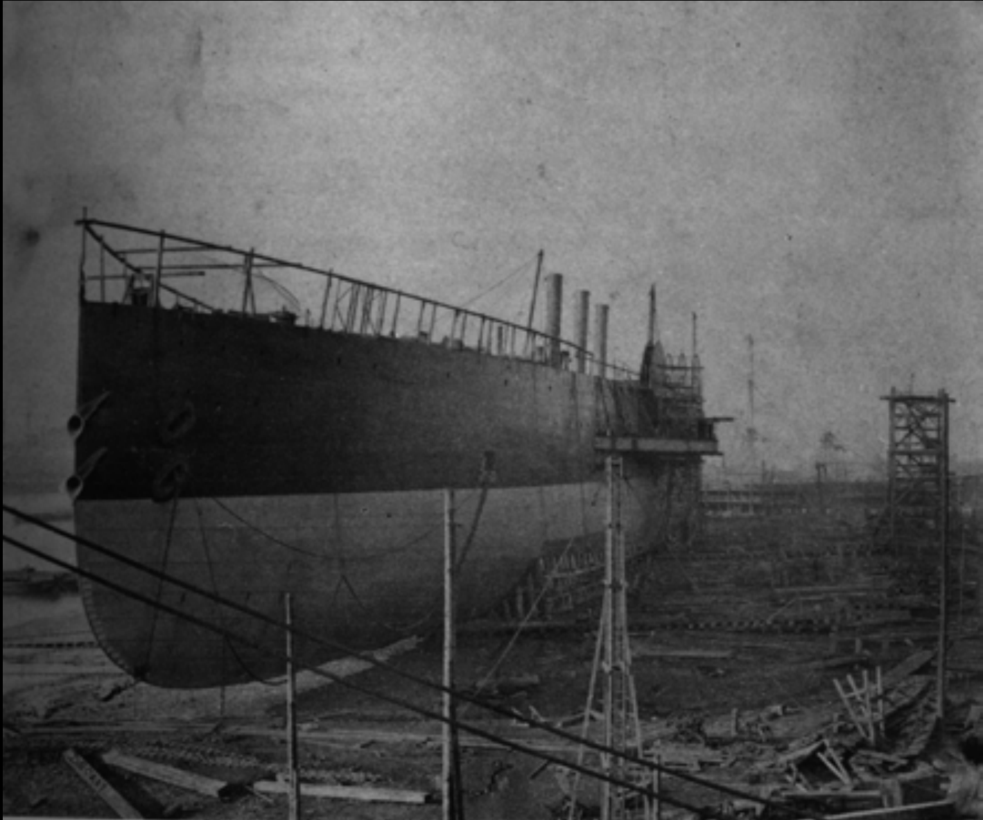
Robert Howlett, The Great Eastern Under Construction , 1857
